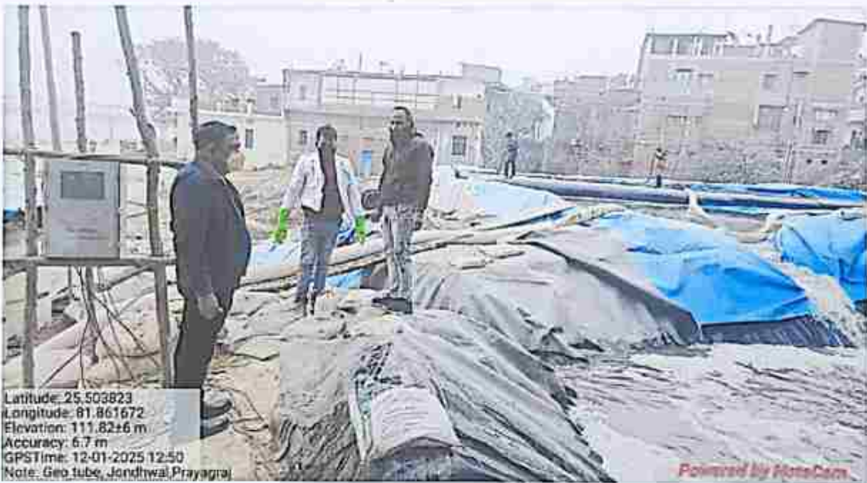
Geo Tube Treatment, Jondhwal Drain, Prayagraj
