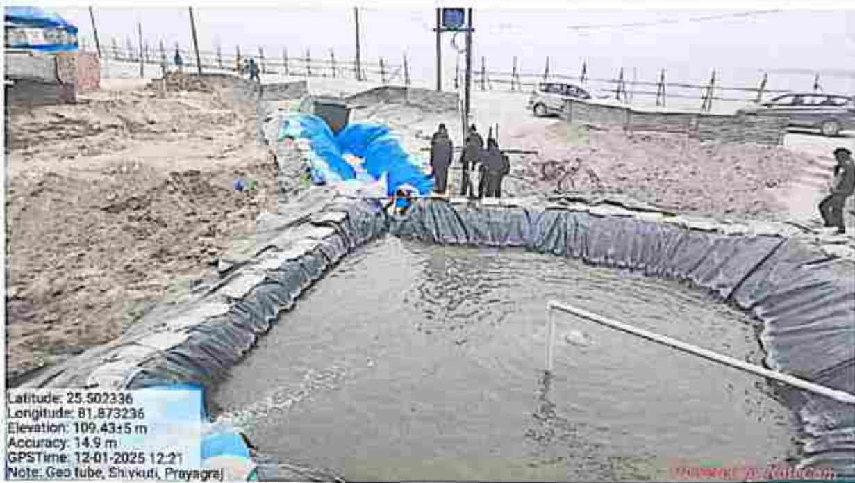
Geo Tube Treatment Shivkuti Drain, Prayagraj
