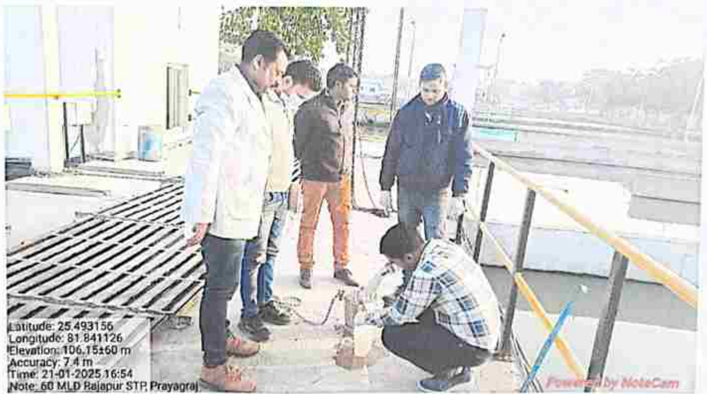
60 MLD, STP Rajapur, Prayagraj
